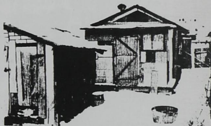
This house is condemned, but, because they are Negroes, this Erie family must live in this dwelling —
