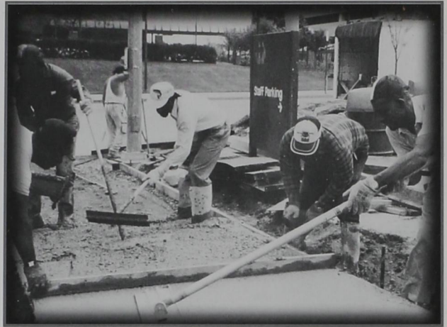
Courtesy of Crenshaw Brothers Construction The hiring of minority contractors and laborers remains an issue in the 1990s. A Crenshaw Brothers Construction crew at work at Hamot Hospital.
